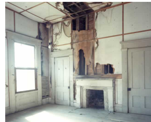
TOP LEFT: The central hallway before restoration work began. Shattered plaster is visible and fallen ceiling pieces were replaced by wooden boards.
